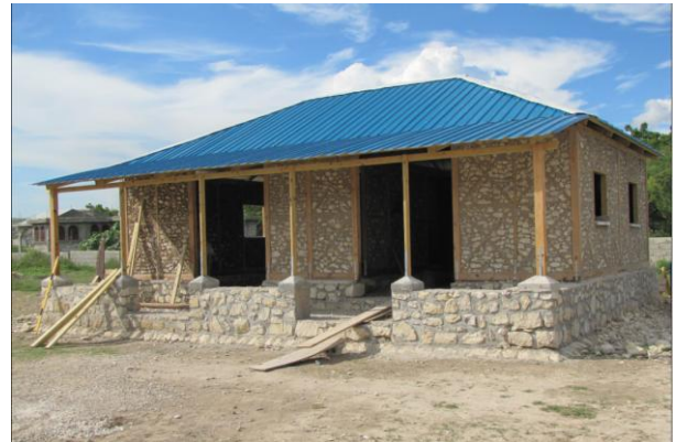
A community building built in Camp Corail with debris generated by the earthquake. Photo credit: Entrepreneurs du Monde
